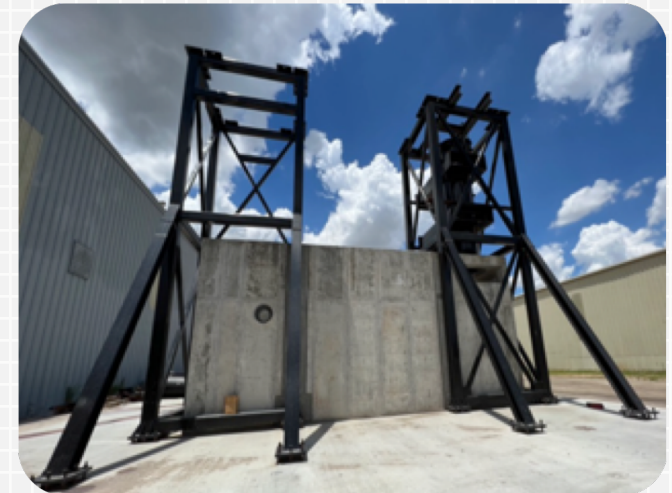
Genergy Hydro Electric Power Tower Under Construction in Houston
